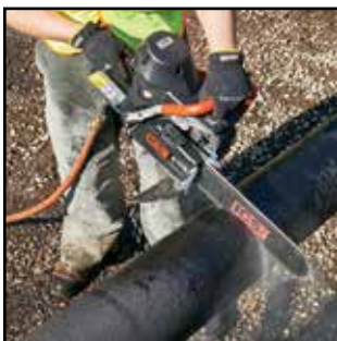
Cut up to a 25cm (10 inch) pipe from one side.
